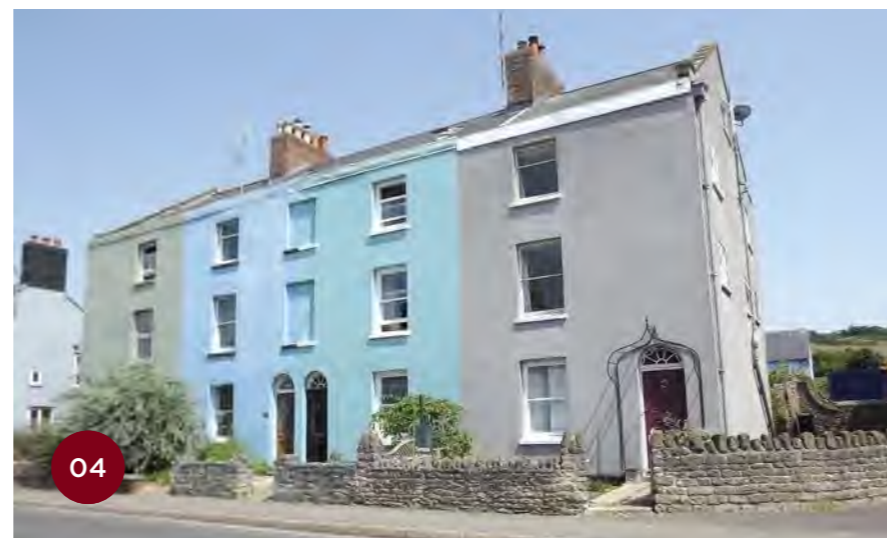
04 Natural colour and painted render finish used along brick chimneys and slate roofs.
