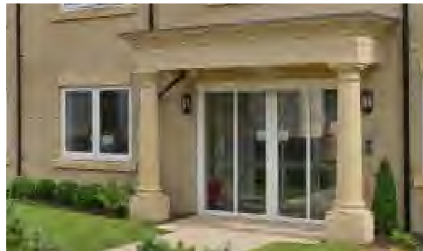
3. Entrance Canopy - Cast Stone Traditional Portico
