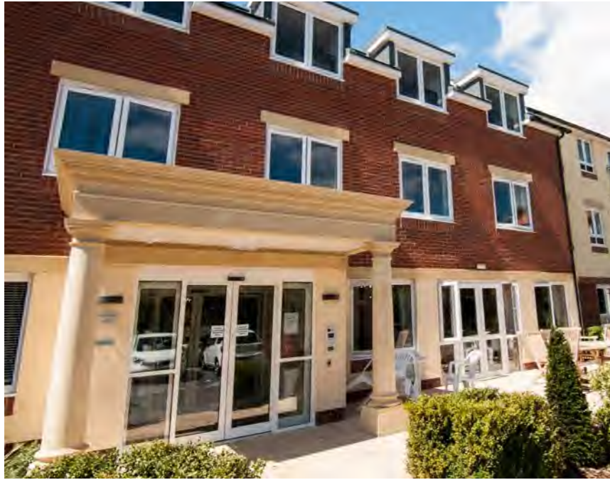
Secure Main Entrance from Parking
