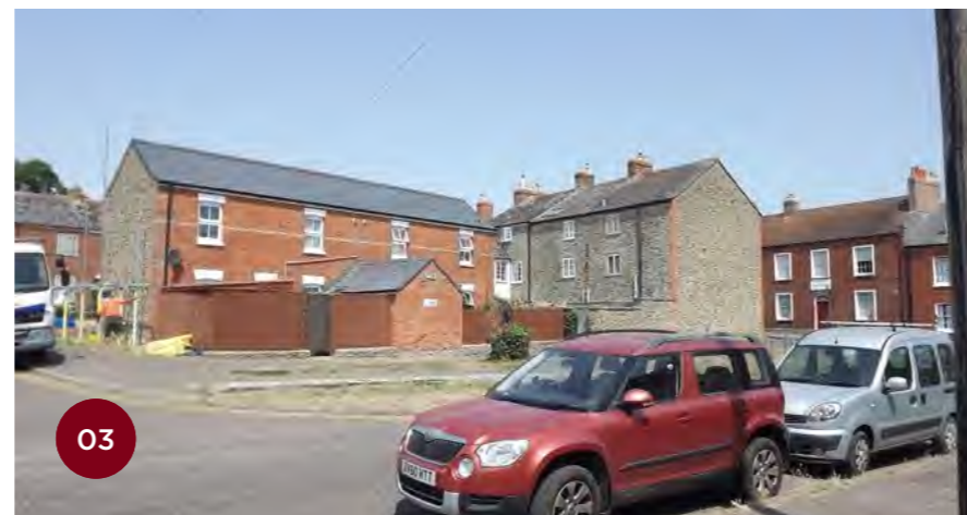
03 Coursed rubble stone properties, with stone and brick detailing in between brick properties.
