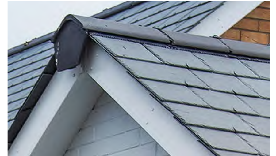
5. Slate Roof with white uPVC Fascias and Soffits
