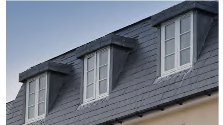
6. Dormer Windows - Stormking lead-effect GRP dormers with white uPVC windows inset.
